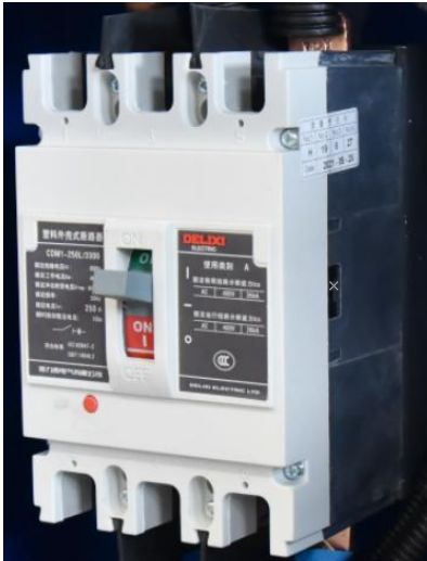
Figure 7.5 Manual Main Breaker
